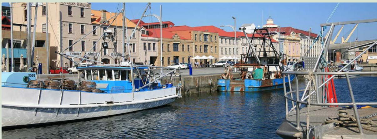
Hunter Street, Hobart. The Tasmanian Heritage Council has determined that more than 70 per cent of the places on the Tasmanian Heritage Register will remain protected and managed at the state level
