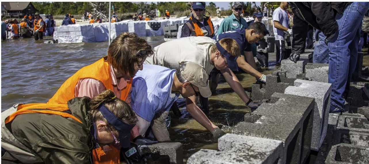
Hundreds of volunteers repair an oyster reef for shoreline protection in the United States. Similar large-scale projects are possible in Australia Photo by Erika Nortemann, © The Nature Conservancy
