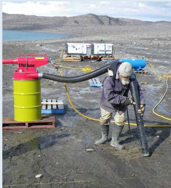
Vacuuming contaminated soil from the Lake Dingle spill
