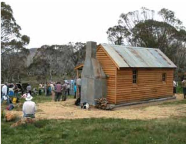
■ The Broken Dam Hut re-opening, December 2007, Kosciuszko National Park, New South Wales Photo by Geoff Ashley
