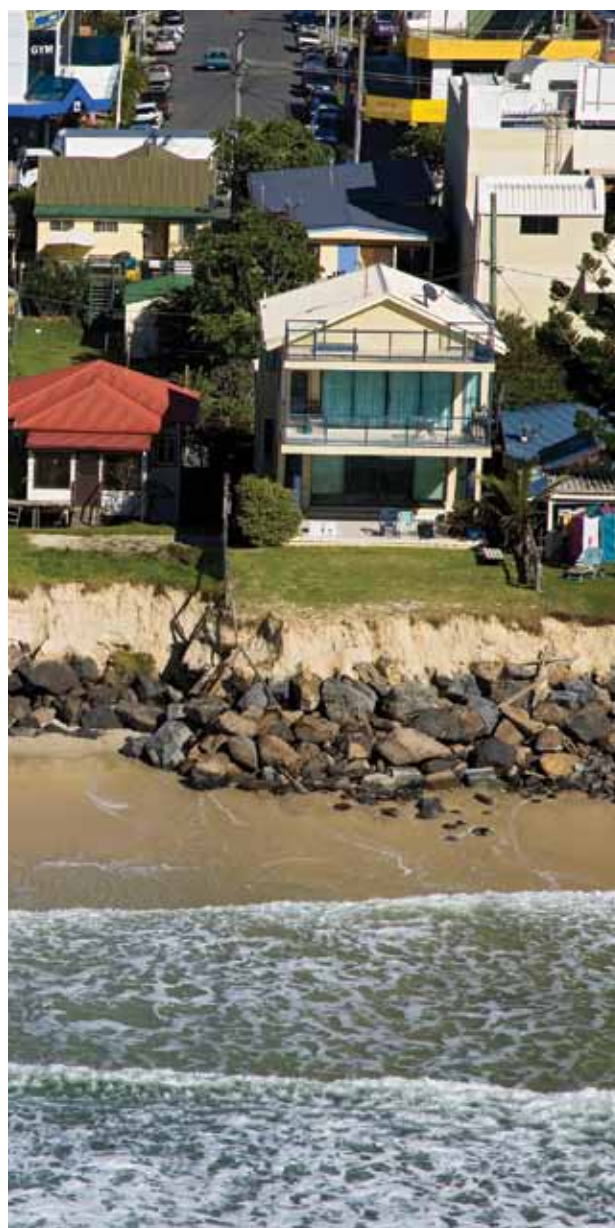
■ Beach erosion following storms in May 2009, Palm Beach, Queensland Photo by Skypics
