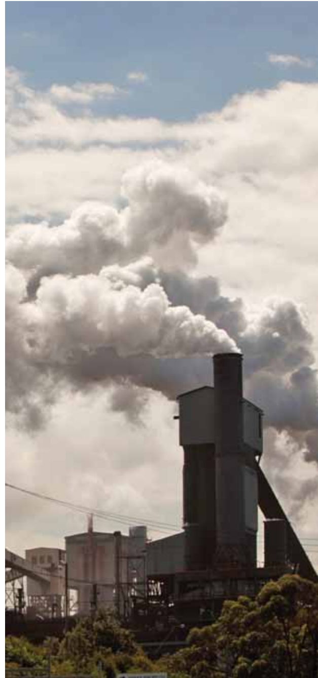
■ Emissions from the steel works at Port Kembla, New South Wales Photo by Ashley Cooper
